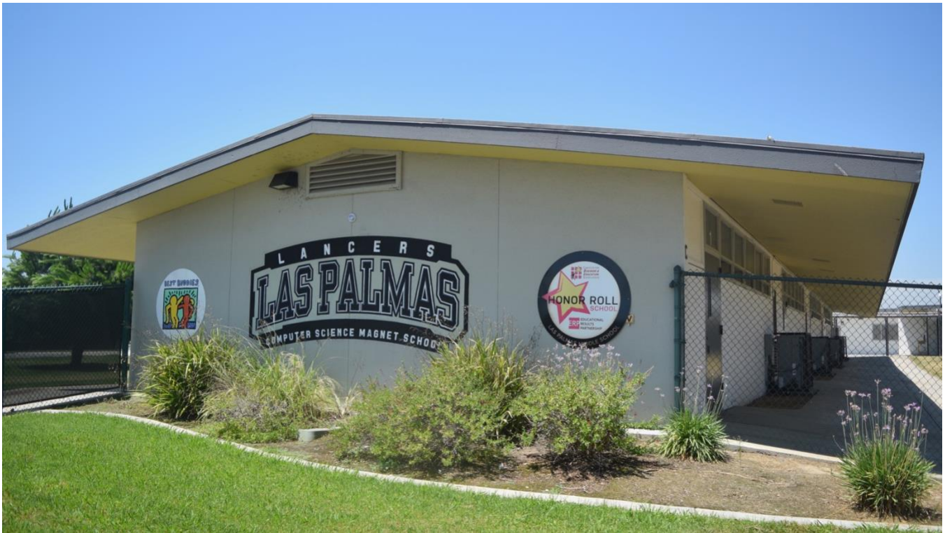
CVUSD_ENERGYSTAR2: Las Palmas Middle School earned ENERGY STAR Certifications by meeting ventilation standards set by the United States Environmental Protection Agency and rating in the top 25 percent nationwide for energy efficiency.
