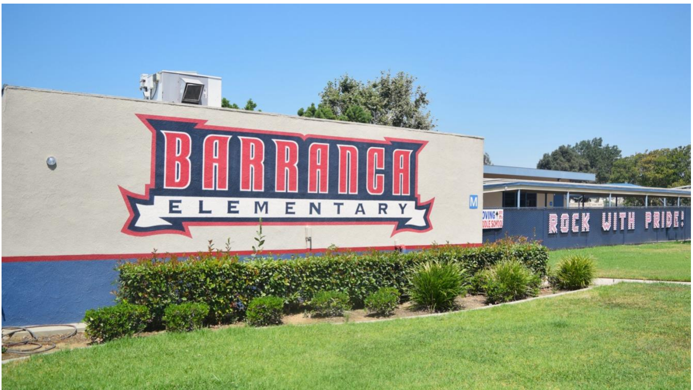
CVUSD_ENERGYSTAR3: Barranca Elementary School was one of 12 Covina-Valley Unified School District schools to receive ENERGY STAR Certification from the United States Environmental Protection Agency.
